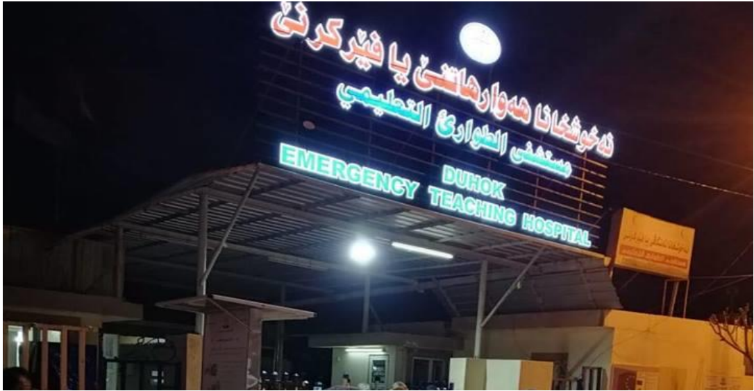
Duhok Emergency Teaching Hospital
